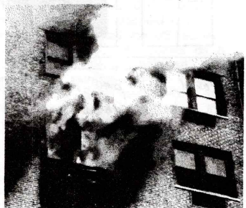
December 29th fire at the Edison Apartments
